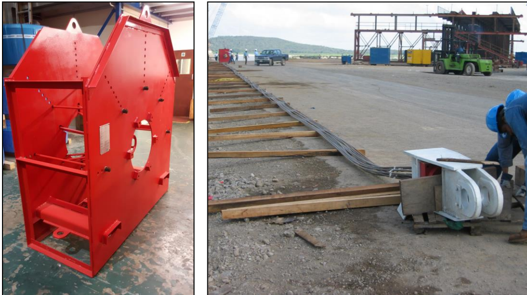
Photos showing DLT strand dispenser and strand pulling/cutting process
